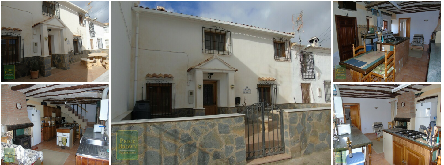
Cortijo Josefina - A village house in the Albox area. (Partially Reformed)
