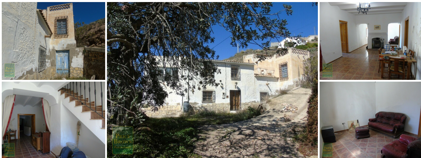
Casa Cueva Mojon - A country house in the Albox area. (Partially Reformed)
