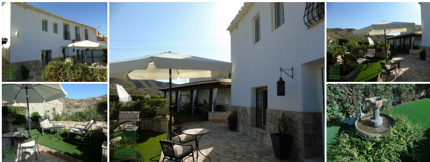
Casa Lynda - A country house in the Arboleas area. (Renovated)
